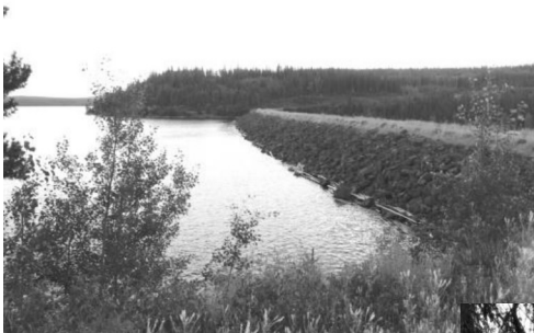
Kenney Dam Site
